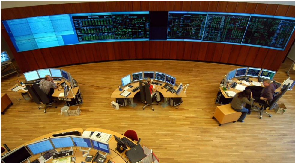
Fig. 7. Large display walls have a great impact on the control room layout.
